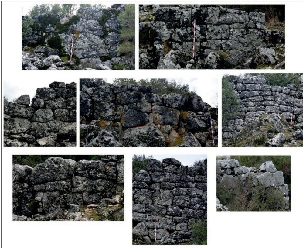
Figür 29. Keraitai, duvar örgü tipleri / Ceraitai, masonry types.
