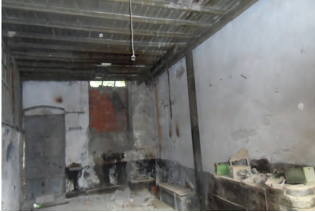
Fotoğraf 16 - Buhar makinesinin bulunduğu Z05 Makine Dairesi / Engine room where steam engine was located in
