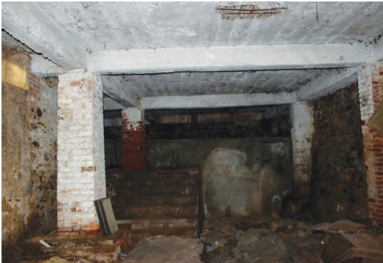
Fotoğraf 26 - B01 Depoda tuğla ayaklar ve merdiven, betonarme havuzlar / Pillars made of brick and stairway, concrete pools in B01 Storage
